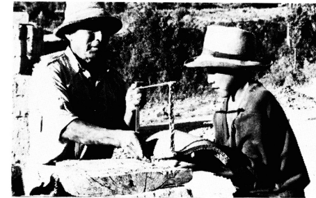
89. Eugenio and aid, making roof tiles.
